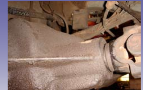
An oily differential housing indicating a leaking pinion oil seal
